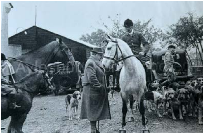
Berkeley Beagles at Great Kimble, October 1945
