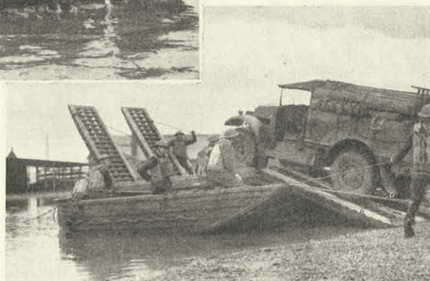
ROYAL ENGINEERS AT WORK — A pontoon raft coming ashore after ferrying a mechanised transport unit across a river, and (right) method of loading lorries aboard a tracked raft for ferrying
